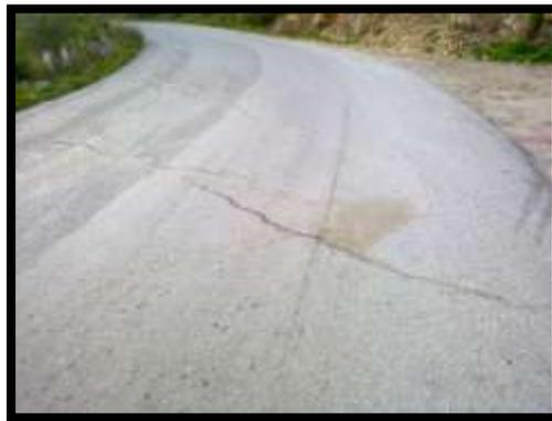
**Fig. III.34: Fissures transversales. RN 71 (ASSIF USSERDOUNE)**
