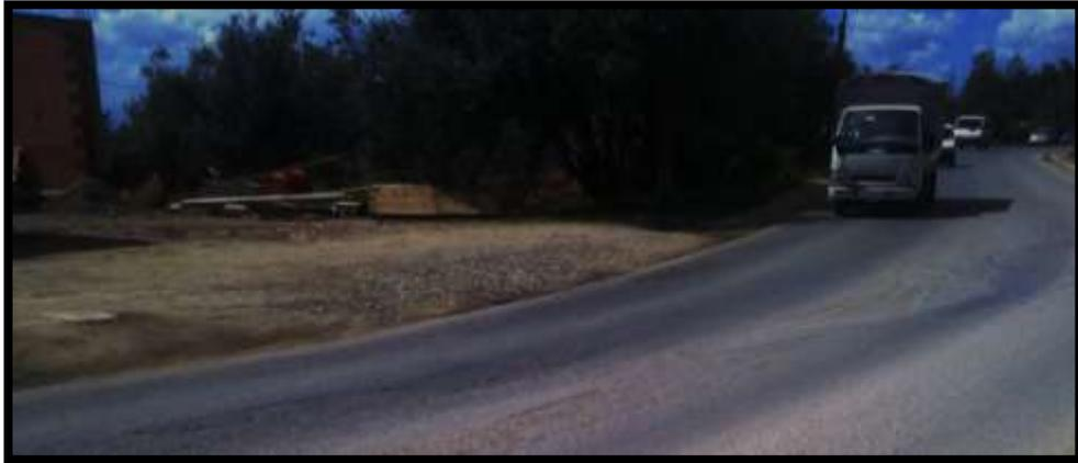
**Fig.III.46: Ressuage. RN 71 (CHEURFA)**
